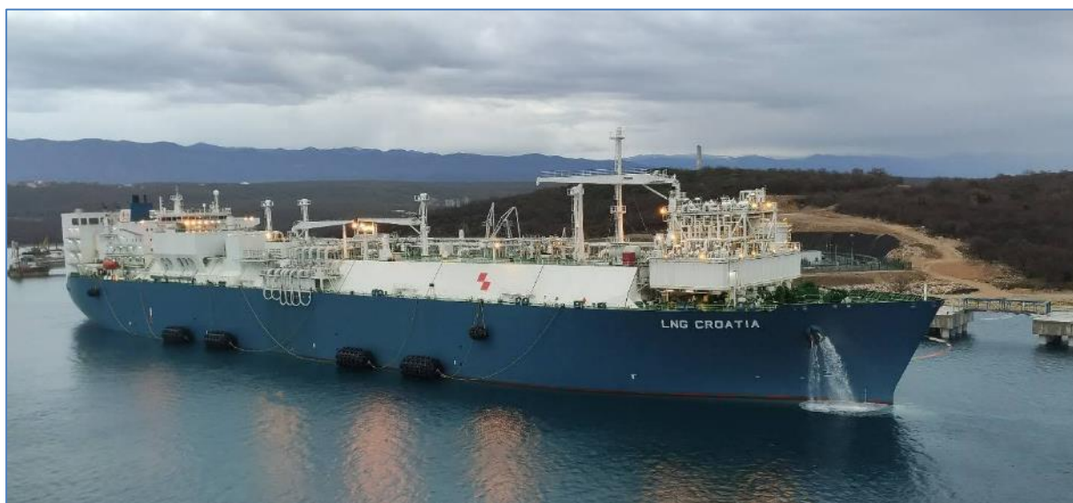
Figure 30 FSRU “LNG Croatia” with “Yokohama” fenders on the LNG ship berthing side
